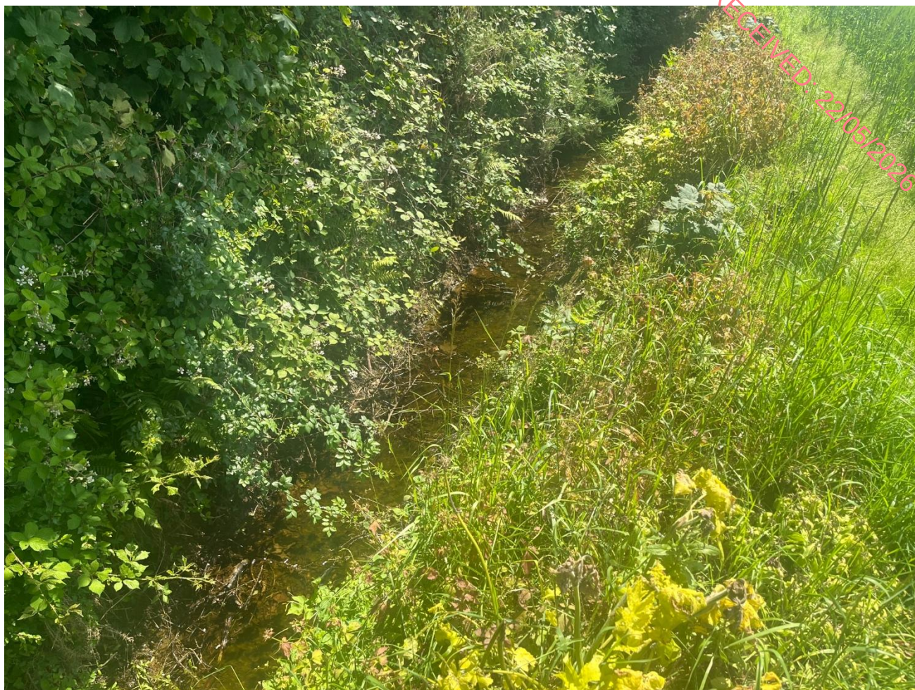
Figure 11: Flooded drainage ditch running along the site boundary
